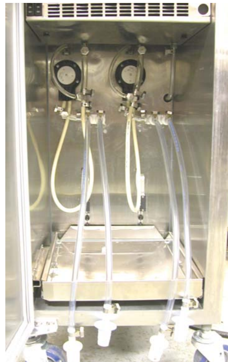
Figure 2-7 Completed BCS Hose Assembly
